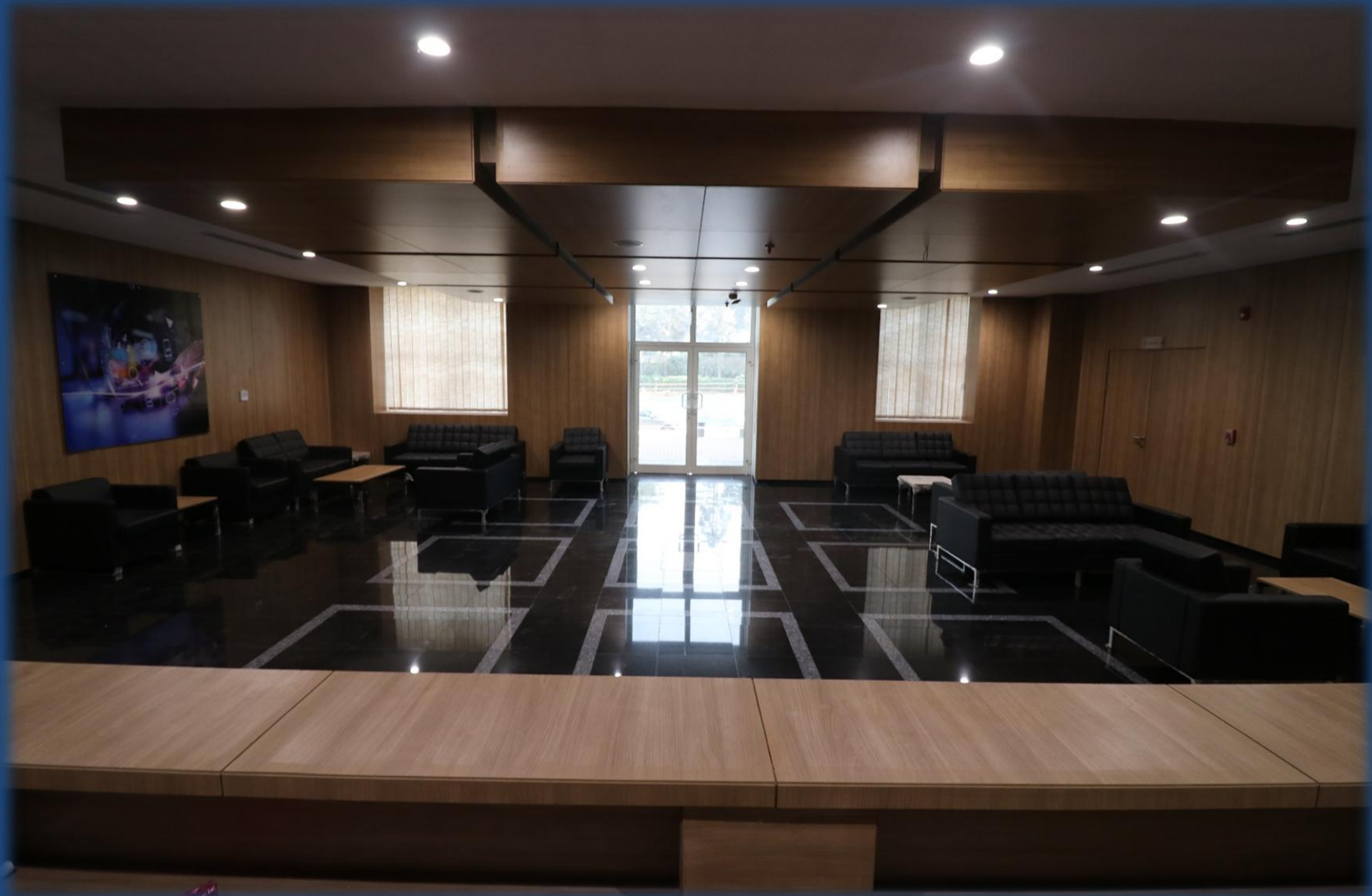
Data Center – Ain Shams University
