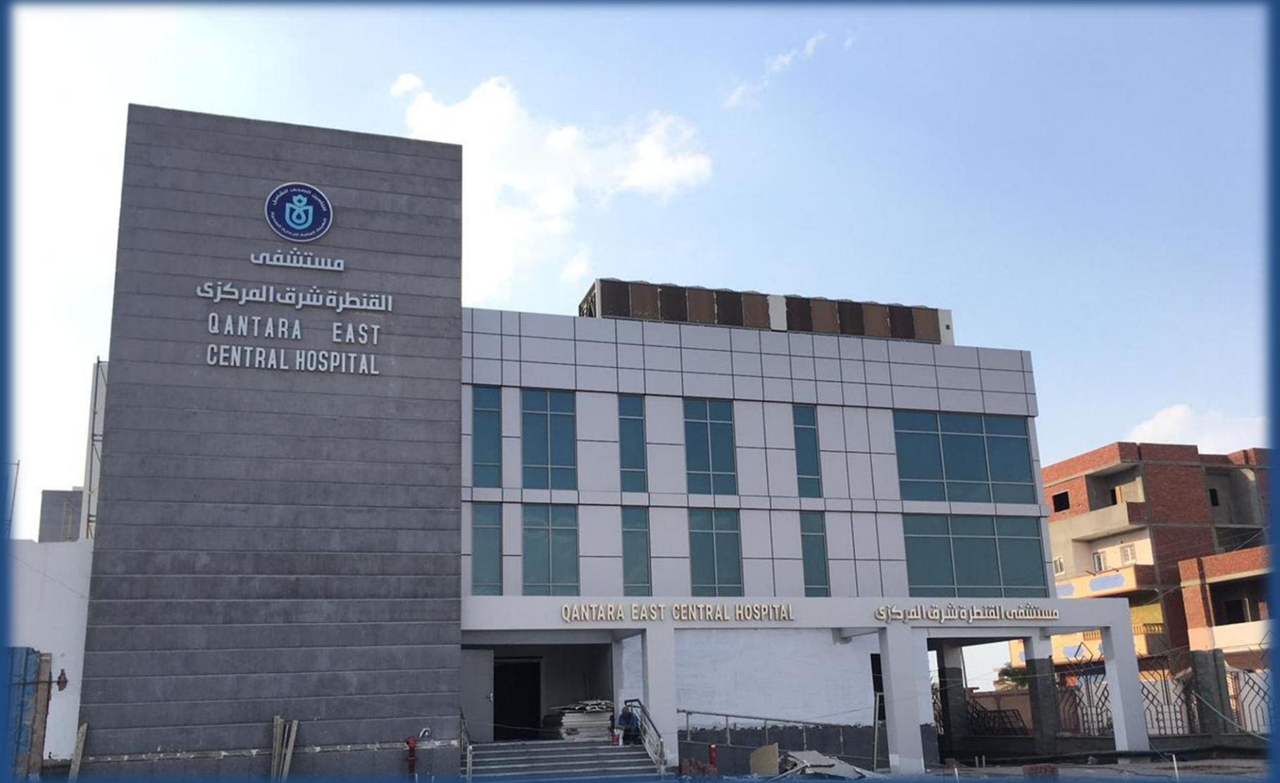
Qantara East Central Hospital
