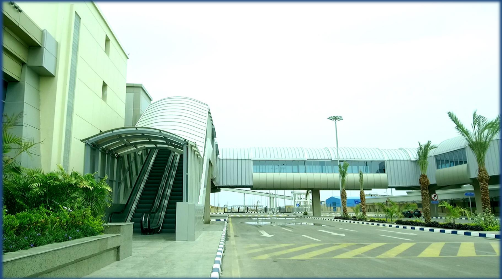
Bridge between arrival and departure Terminal – Safaga Port
