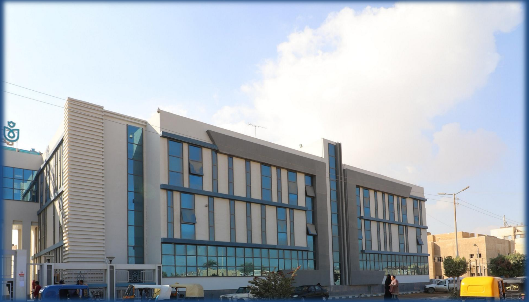
Fayed Specialized Hospital
