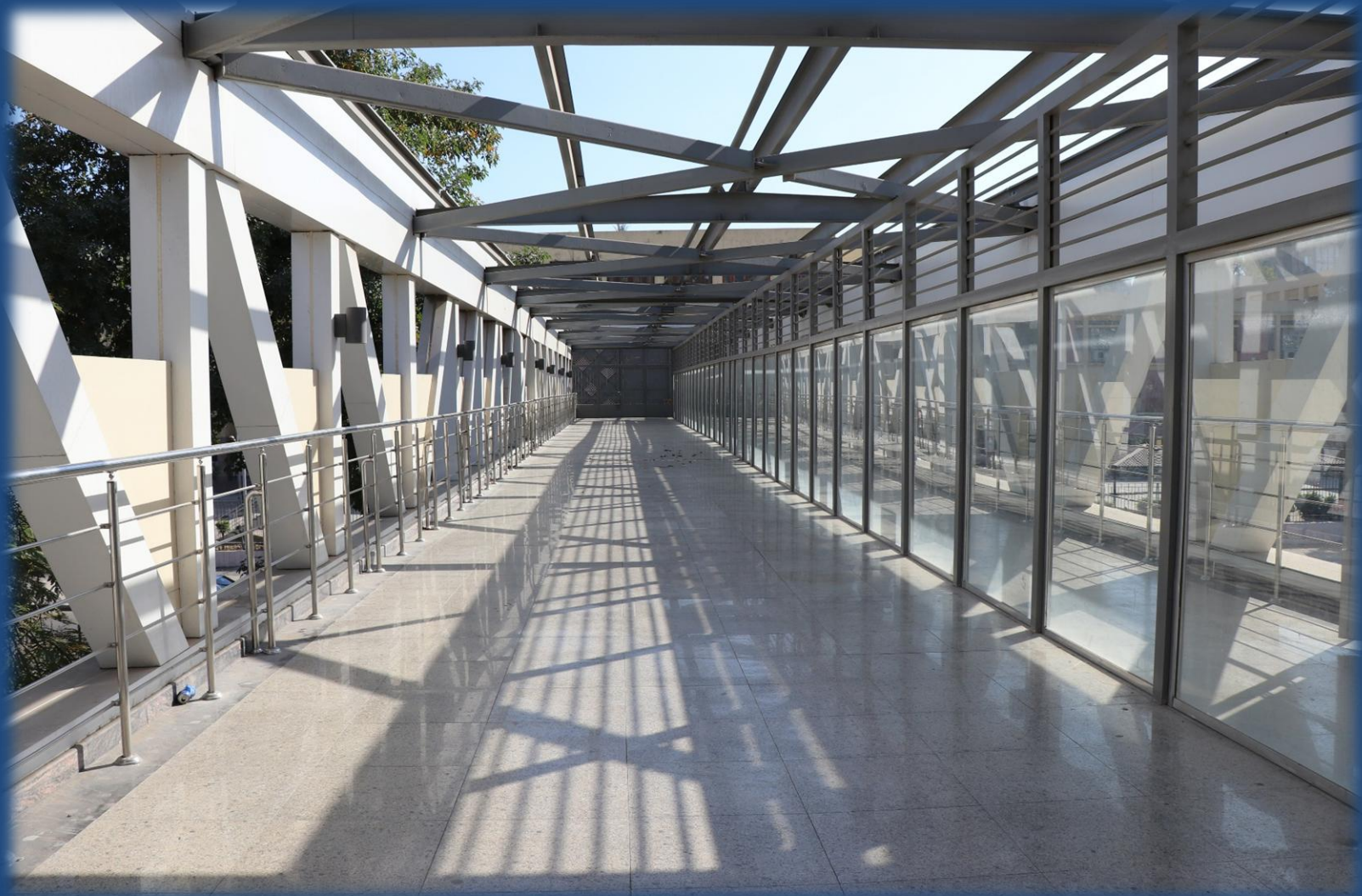
Pedestrian Bridge – Ain Shams University
