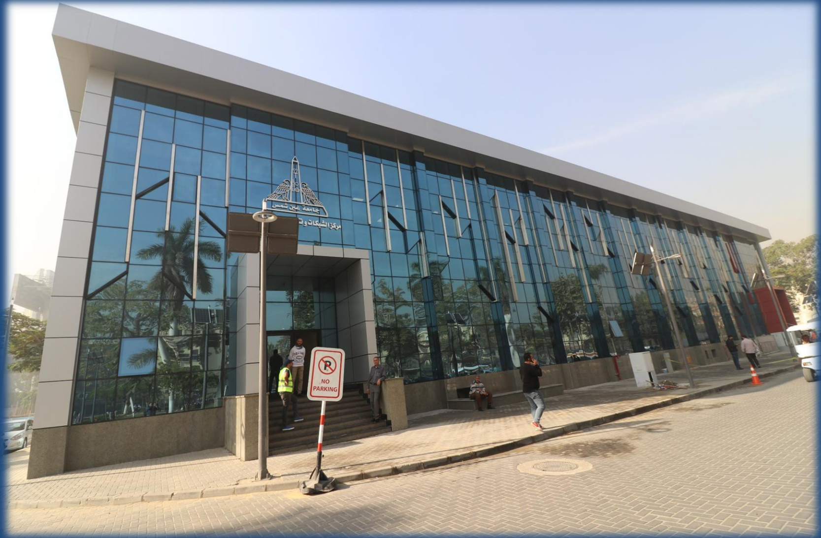
Data Center – Ain Shams University
