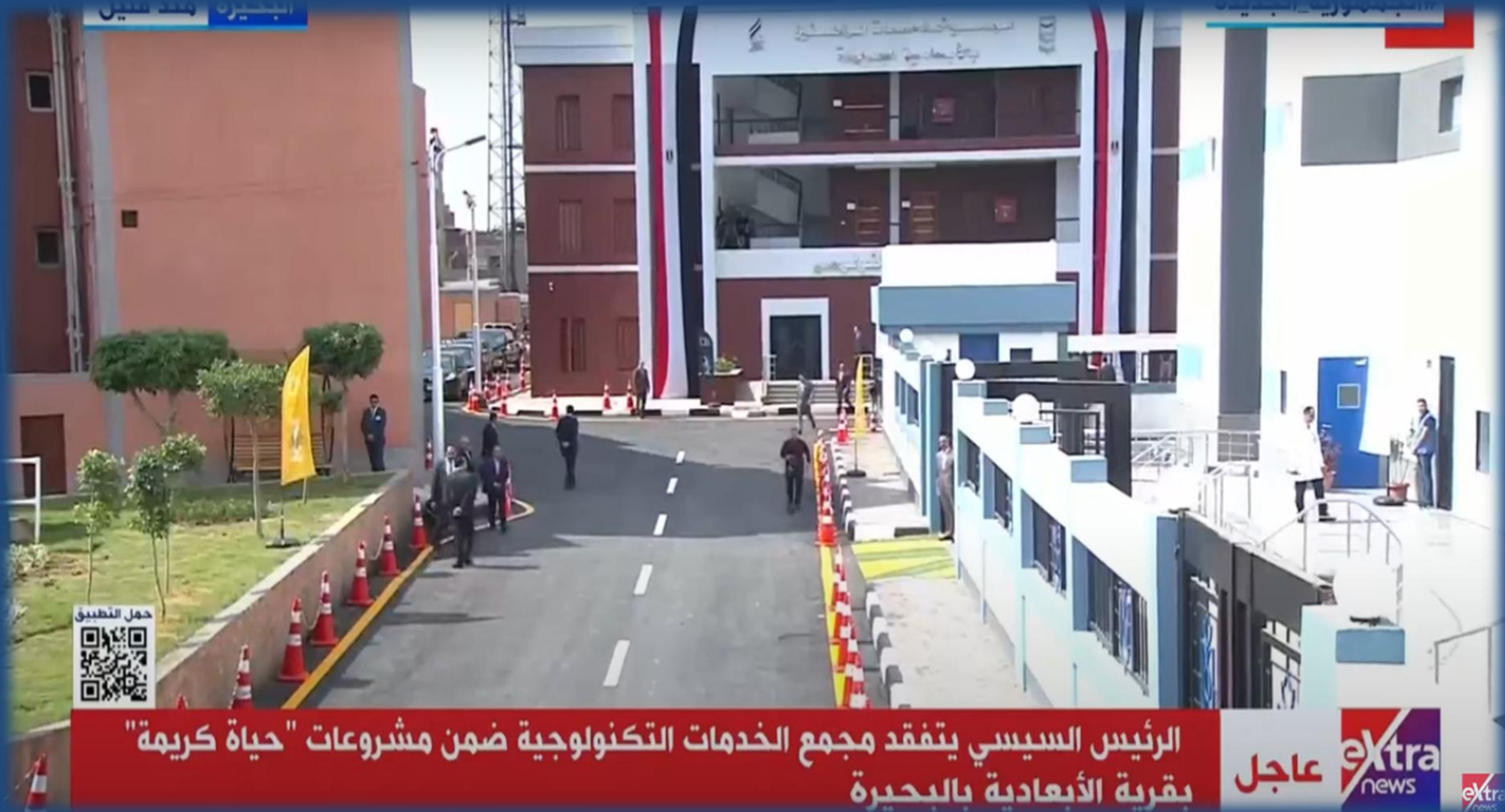
The presidential opening for Al-Abadia Administrative building - Al Beheira Governorate
