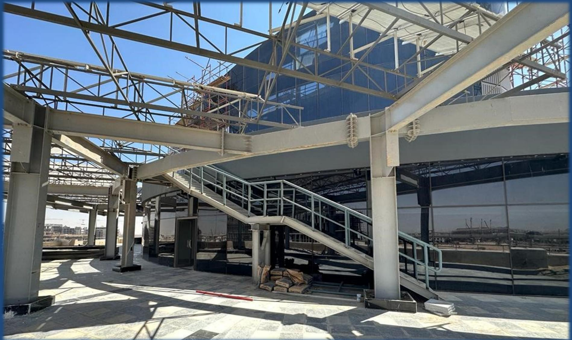
Steel Work – Post Office Headquarter in New Administrative Capital
